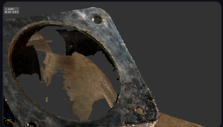
Close up on a flange face and bolt hole, straight from the imager.
